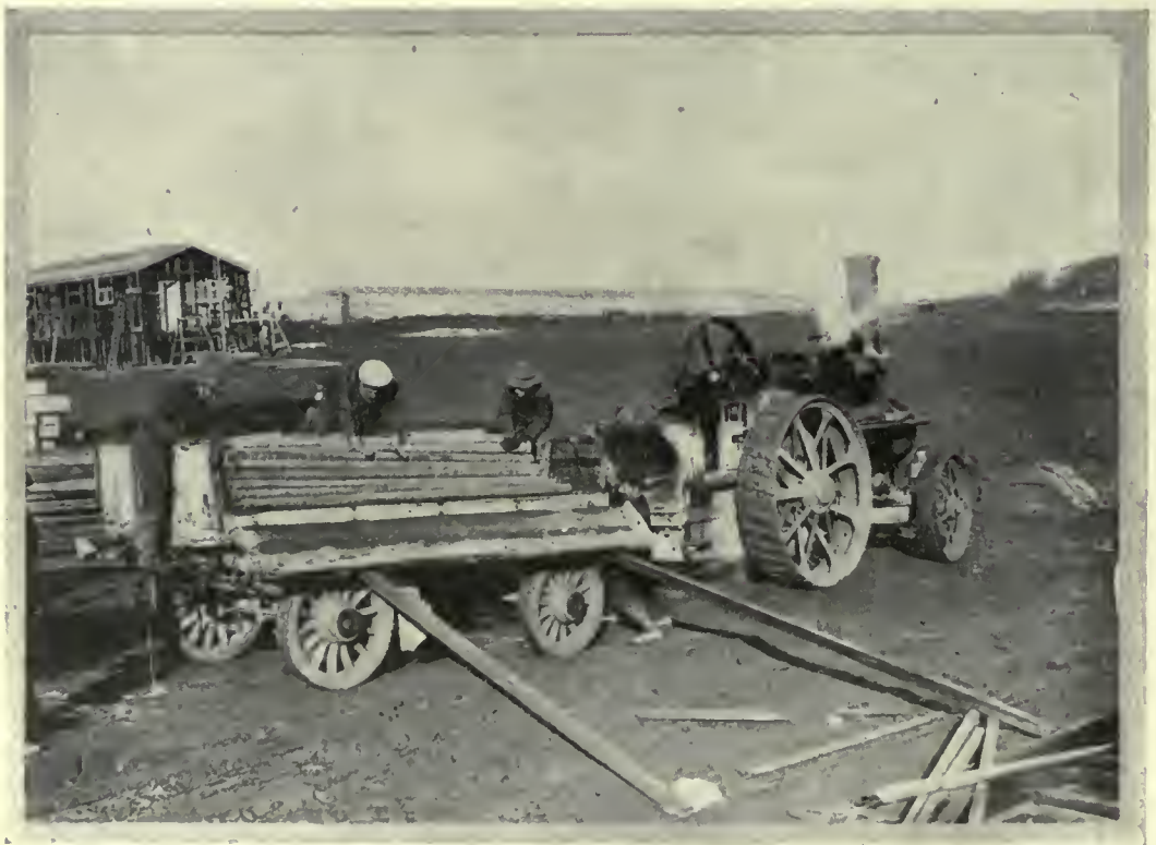
BIRMINGHAM BOY SCOUTS BUILDING HUTS FOR THE WAR OFFICE. Unloading uprights.
