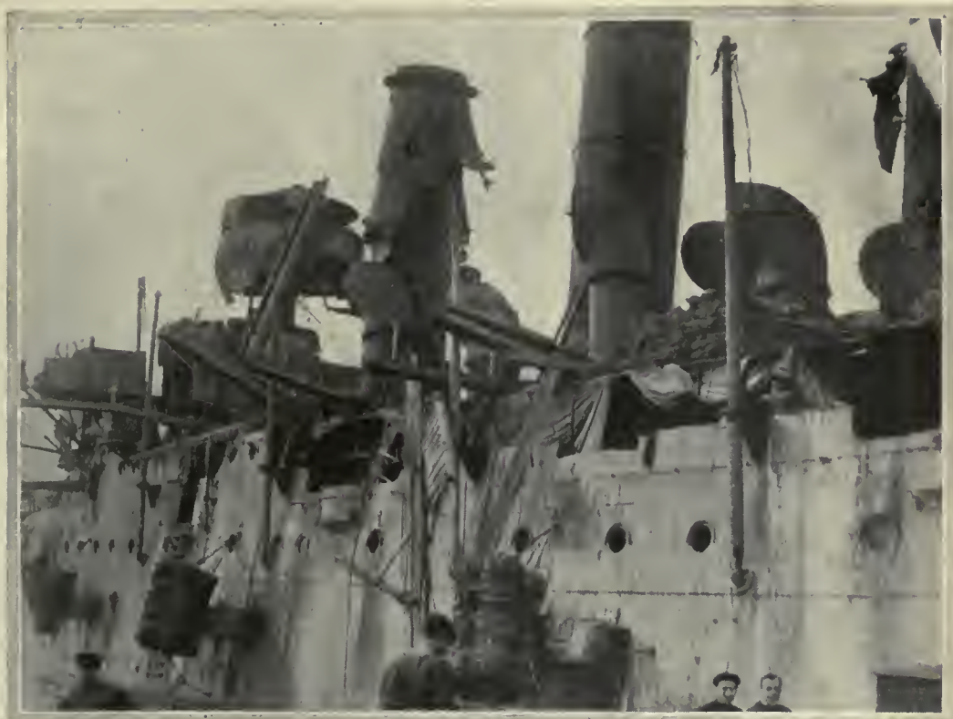
THE VINDICTIVE, PHOTOGRAPHED ON HER RETURN FROM ZEEBRUGGE, SHOWING THE IMPROVISED "BROWS" USED FOR LANDING ON THE MOLE.
