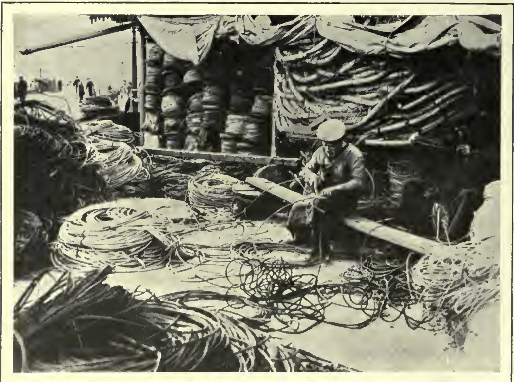
SPLICING WIRE TO BE USED FOR NETS.
