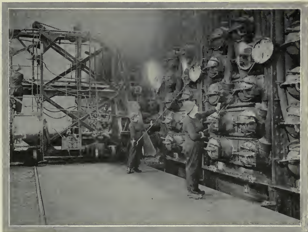
MECHANICAL DISCHARGE OF HORIZONTAL RETORTS.
