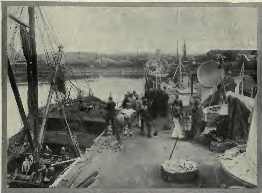
COALING A WARSHIP FROM A LIGHTER ALONGSIDE.
