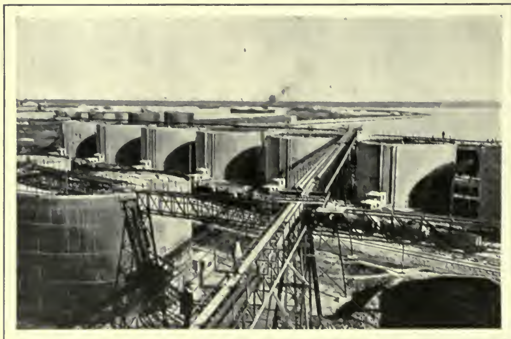
PETROLEUM TANKS AND DOCK, CONSTANZA.
