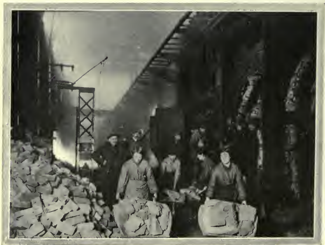
REBUILDING FIRECLAY RETORT BENCHES.
