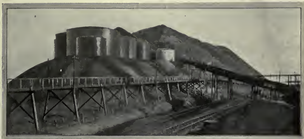
HILL OF SPENT SHALE, WITH STORAGE TANKS.
