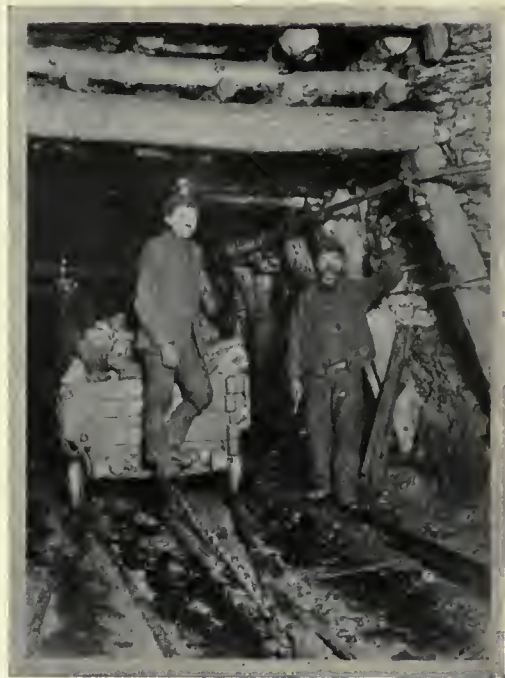
A MINE "ROAD," Showing method of propping the roof, and chain for hauling the trucks.
