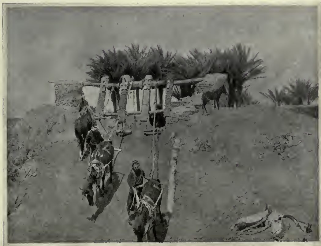
A TYPICAL "WATER LIFT" IN MESOPOTAMIA. This particular example was photographed at Ctesiphon.
