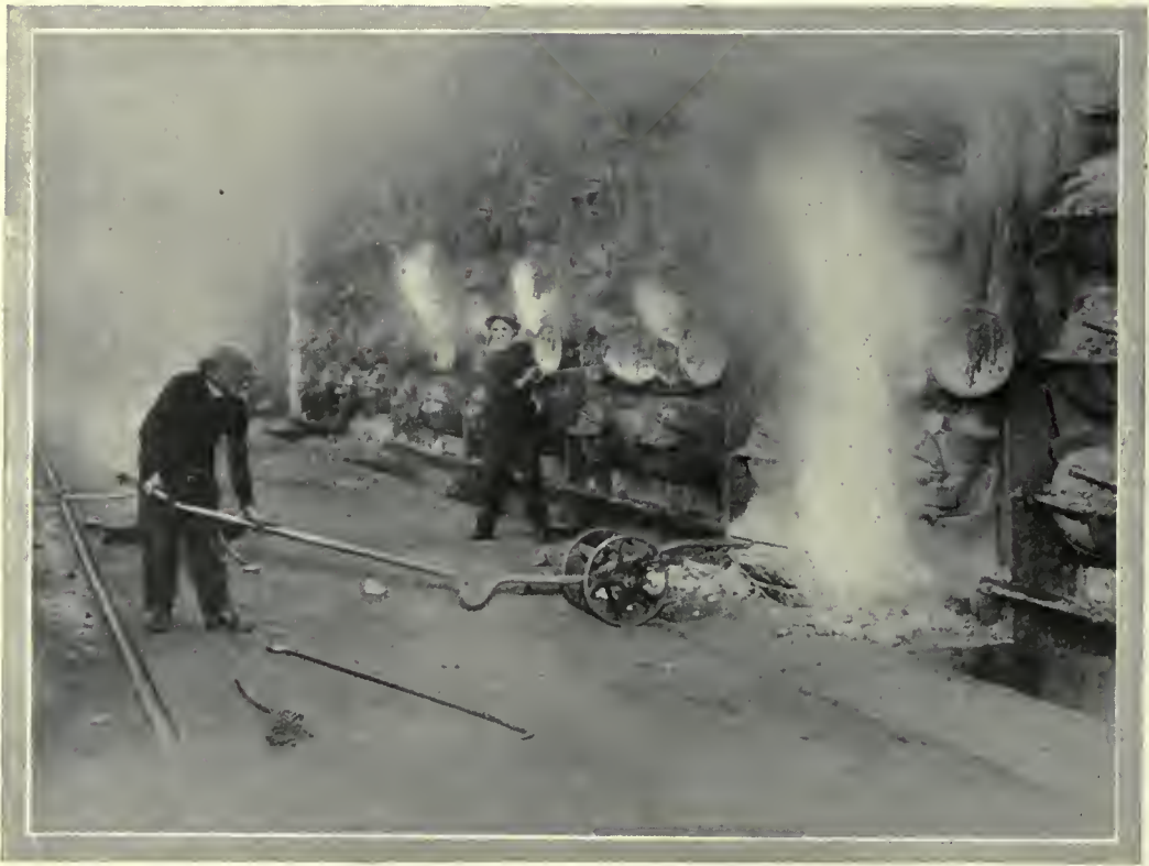
HOT WORK WITH A GAS RETORT FURNACE.
