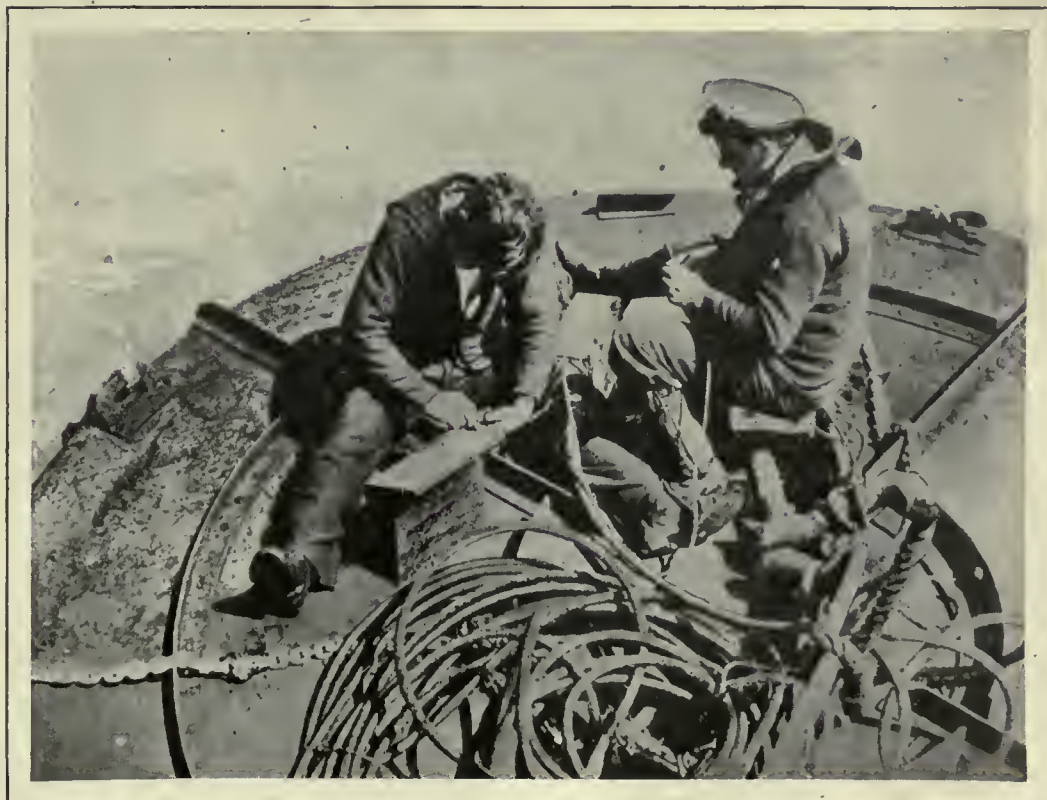
Official photograph. CONNECTING ELECTRIC BATTERIES WHICH FIRE THE MINES WHEN A SUBMARINE IS CAUGHT IN THE NET.
