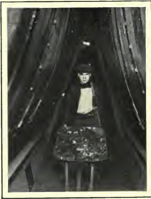
BETWEEN A SHIP'S BOILERS.
